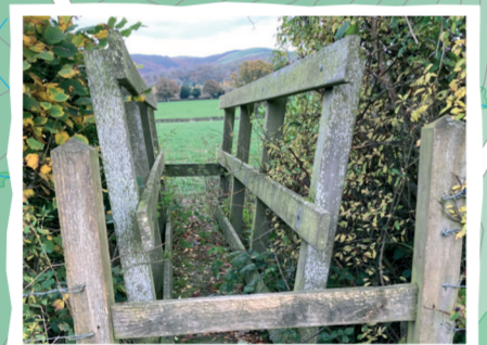
Pont ar llwybr 5. Bridge on route 5.
